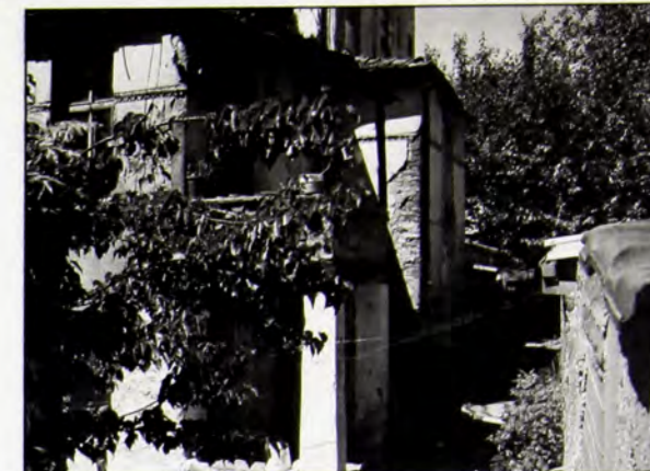
Figure 3 Post-earthquake wooden prefabricated housing in Taftalidz
