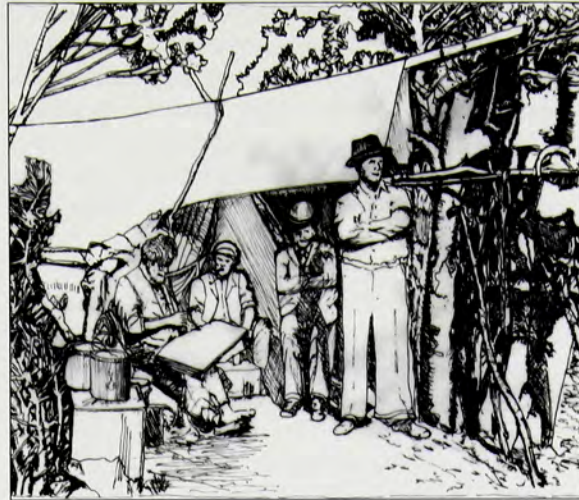
Figure 3 Tent with 'loggia' for breezeway and shade, 1896 Adapted from Battye Library Photograph- 20163P. Illustration by author, 2004
