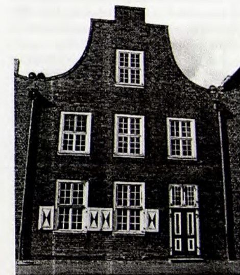
Fig 3: Mittelstraße in the Dutch Quarter (photograph from 2000)
