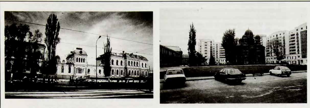
Fig.7. (Left) Brincovenesc Hospital (XIX century) and the church of Dominita Balasa. Photo by Prof. Sorin Vasilescu (early 1980's) (Right) The same area as it is today. The hospital buildings were demolished and the church screened by ten-storey buildings from the Victoria Socialismului Civic Centre. Photo by the author (1992)
