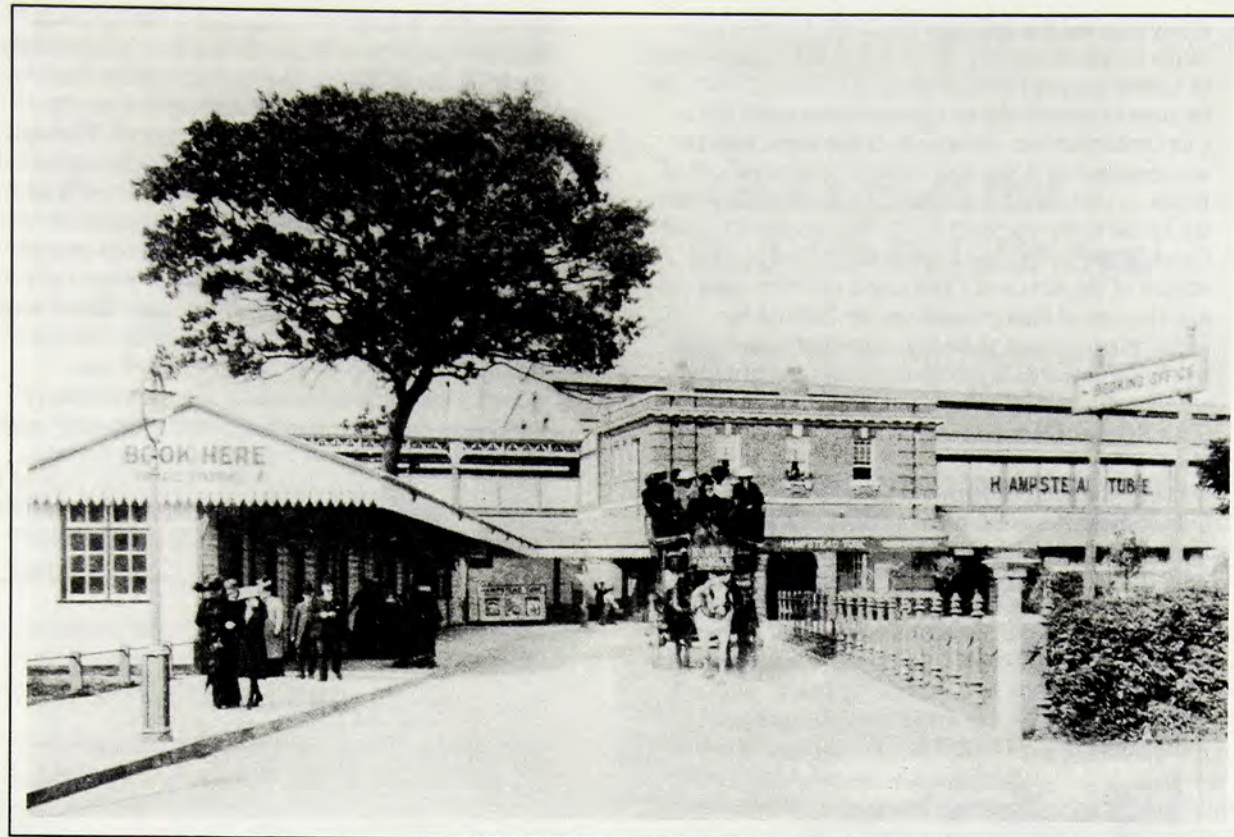
Figure 2: Golders Green Underground Station shortly after opening. (Hampstead Garden Suburb Trust.)
