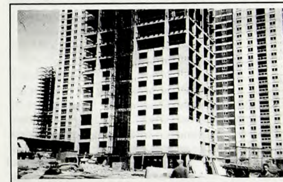
Figures 10 & 11: Red Road development under construction, c1965.
