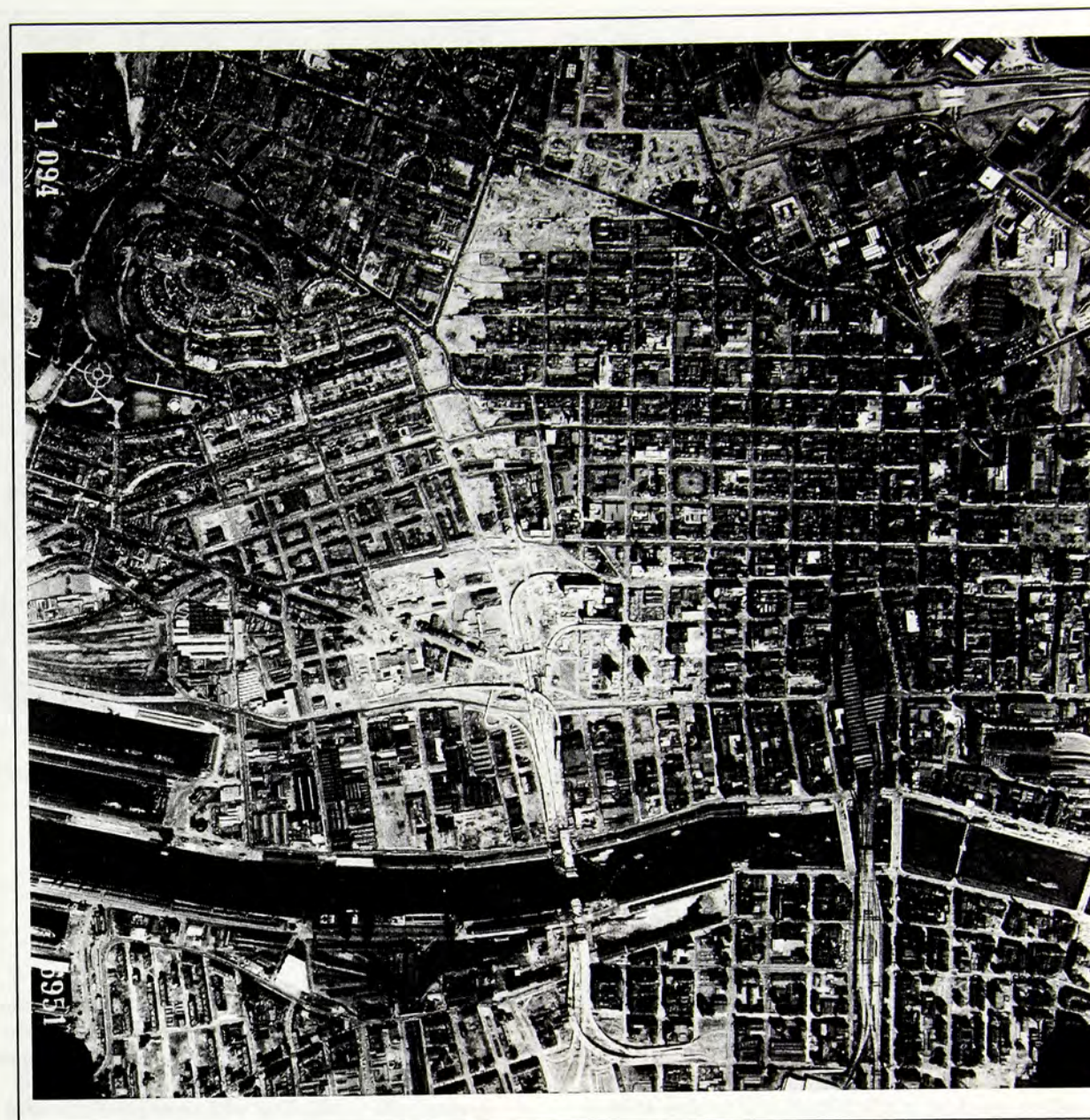
Figure 2: The Glasgow Inner Ring Motorway. Aerial view 1969 showing Kingston Bridge under construction and north flank cleared.
