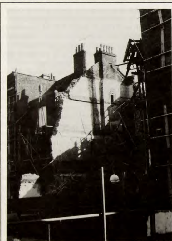
Numbers 47-50 Manchester Street, Marylebone, a 1785-9 terrace, which collapsed during refurbishment in May 1990. Photograph used by Robert Thorne with the permission of the City of Westminster, who called in Alan Baxter & Associates to investigate the cause of the collapse.
